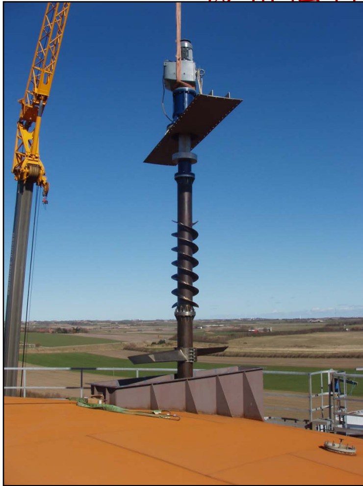
Typical top mounted digester mixer 典型的顶式安装发酵罐搅拌器
