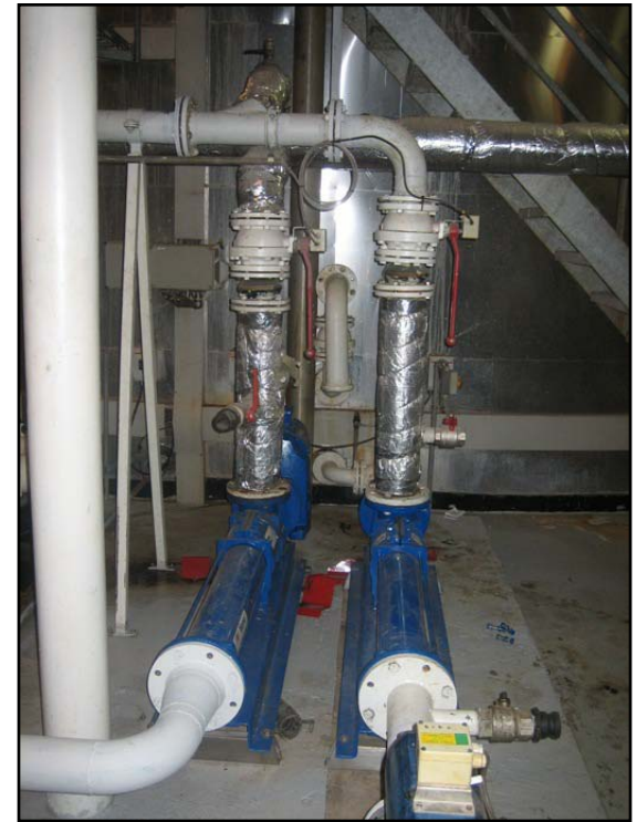
Redundant pump installation 冗余泵系统
