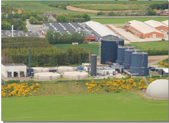
LEMVIG BIOGAS PLANT (1991/92) LEMVIG 沼气厂 (1991/92)
