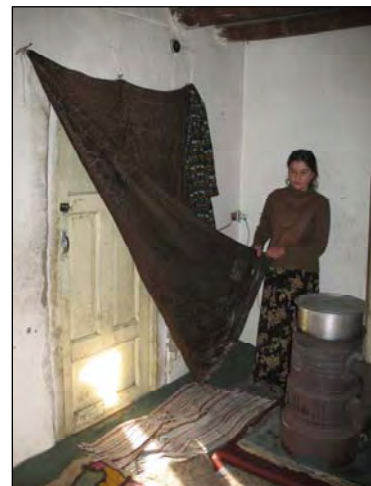
A heavy curtain hanging in front of the door against the wall and to the floor will create an insulating air layer and reduces draft.
