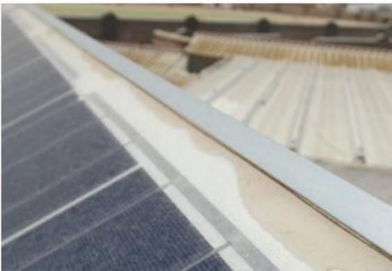
FIGURE 38: DELAMINATION
