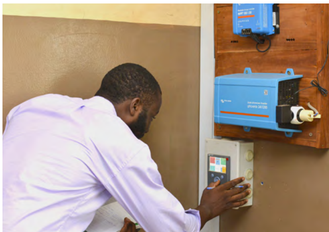
Picture 3: Verification consultant checking the quality of the solar installation
