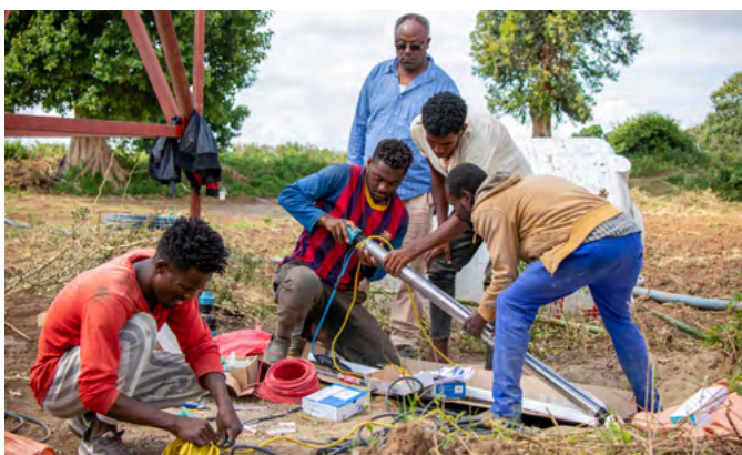
Picture 3: Installation of the solar pumps
