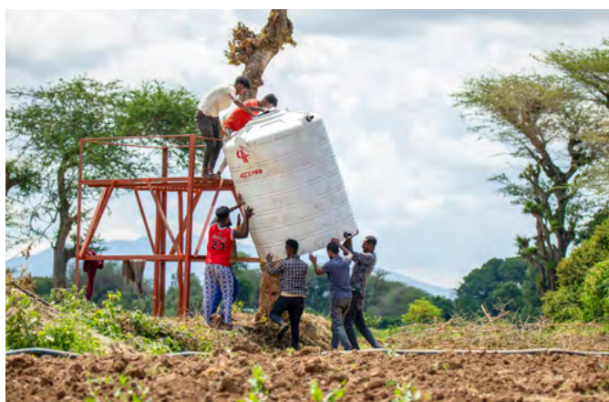
Picture 1: Installation of a water tank
