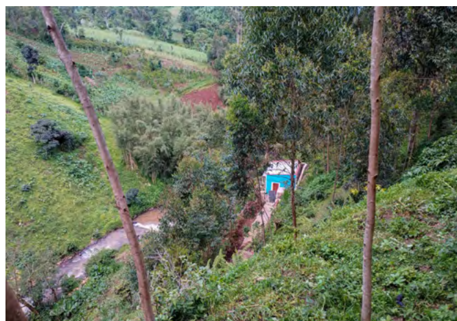
Picture 2: Power block – MHP Gobecho site
