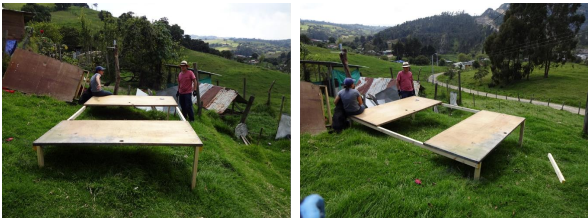
Fig. 19: Topography/slope – wooden construction for PV-structure necessary
