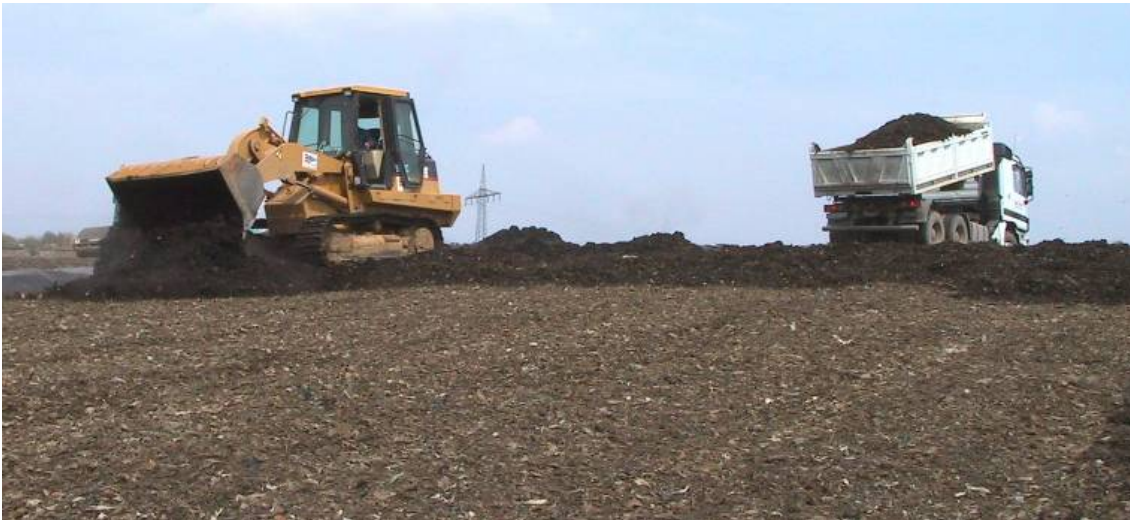
FIGURE 3 Placement on top of a landfill
