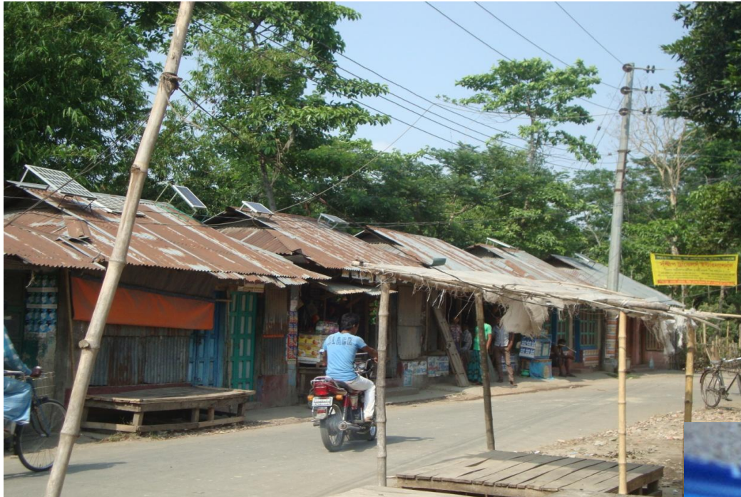
Shops powered by 100 kW p mini-grid and SHS
