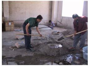
5. First apply a layer (3.5 – 4 cm thick) of the coarse-grained sand-cement mixture on the pile of soil
