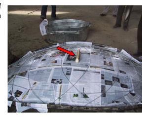
10. Place two welded fastening hooks on the longer sides in the middle between the centre of the form and the flat iron ring.
