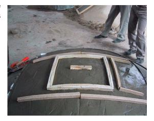
13. The fastening hooks have to be embedded as shown in the pictures to prevent deformation later on.
