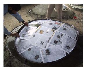
7. Assemble the two parts of the flat iron ring and lay on the form. Then make a mesh from the iron wire and adjust it to the form (see picture).
