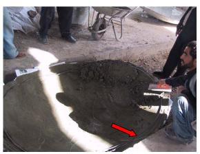
4. Add a 4 cm thick layer of coarse-grained cement Weld four fastening hooks from one flat piece of iron and two iron rods. Press the fastening hooks into the wet cement as shown in the picture and cover it with plastic foil. Let it dry for two days, then remove the plastic foil and sprinkle it with water. Then let it dry for an additional five days.
