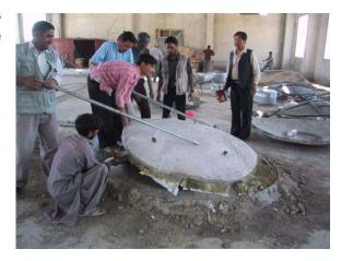
Repair and smoothen the concave curved surface of the master form.
