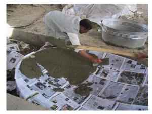
3. Press 14" steel rod into the wet cement at a distance of 5 cm to the edge.
