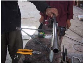
6. The adjusting rod for the solar cooker will be constructed from a U-form made from 2 cm flat iron, a 6cm long piece of pipe with a diameter of 2 cm, 20" iron rod, 8" iron rod and 10" screws as shown in the pictures.
