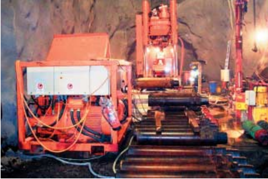
Raise Boring Machine for pressure shaft excavation
