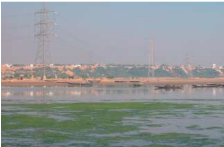
The site for the future Combined Cycle Power Plant Fauji Korangi nearby the city of Karachi
