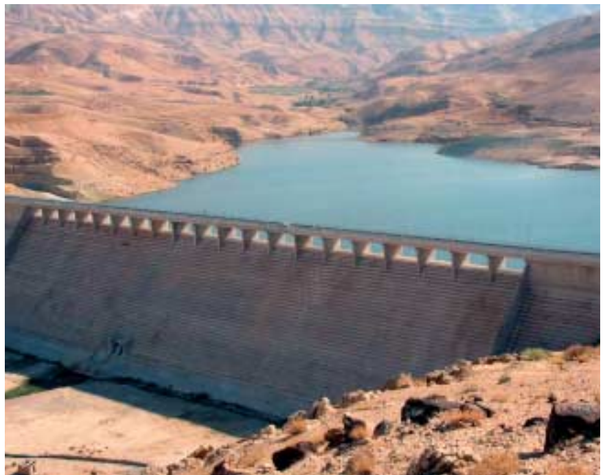
Mujib Dam with partial impounding
