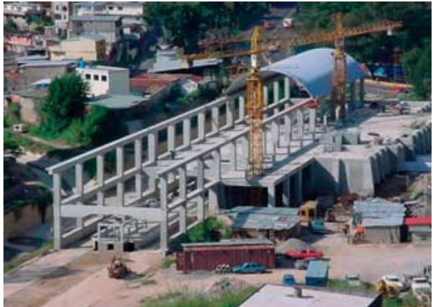
Terminal Los Teques during construction
