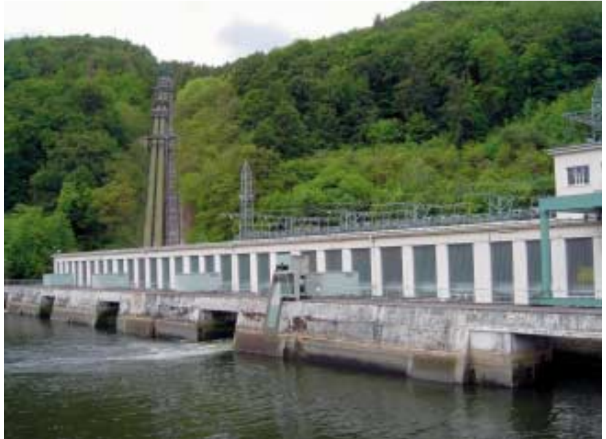
Powerhouse and penstocks of the existing pumped storage plant Waldeck I
