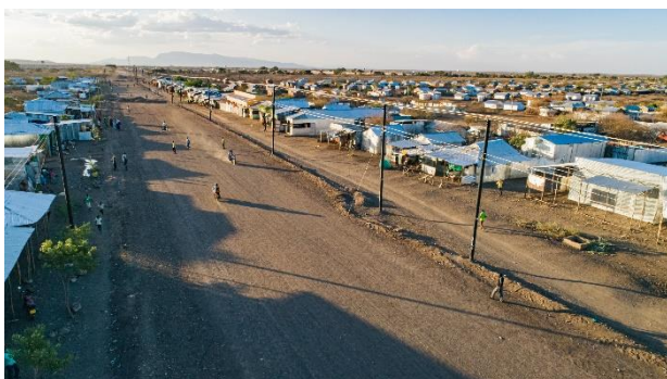
Households, businesses and institutions connected to electricity supply from Kalobeyei settlement mini grid. © GIZ Kenya, 2022
