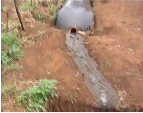
Picture 7: PTD outlet discharging slurry to pit
