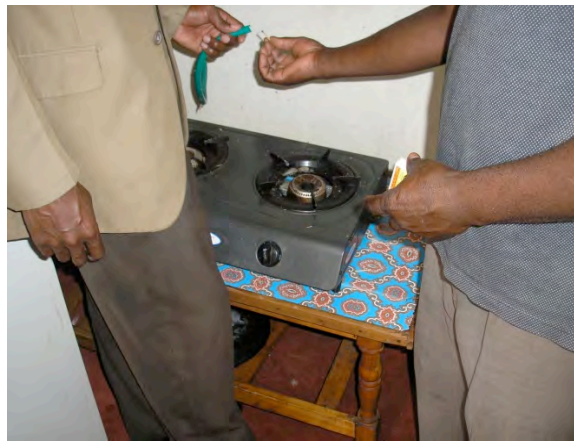
Picture 6: Biogas cook stove, with the feed inlet pipe being shown (Author)
