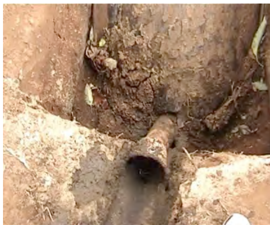
Picture 3: Digester inlet with a trench
