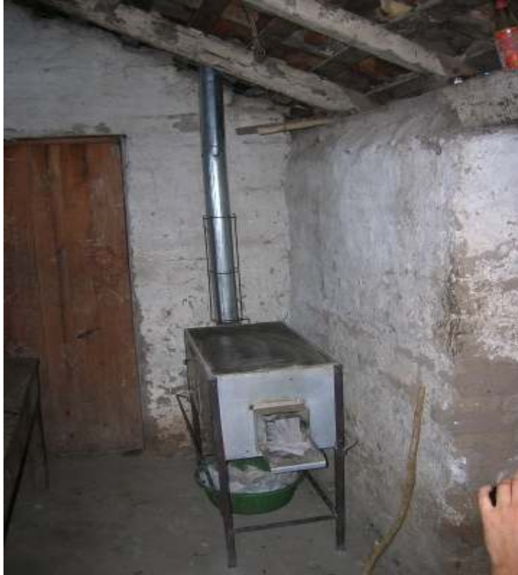
Improved stove (ecofogon) with oven used additionally to the Justa stove
