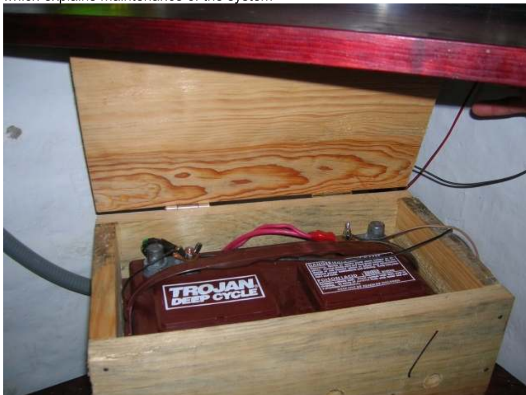
The deep cycle solar battery is delivered in a wooden box for better protection
