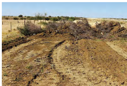
Soil disturbance with grader de-bushing
