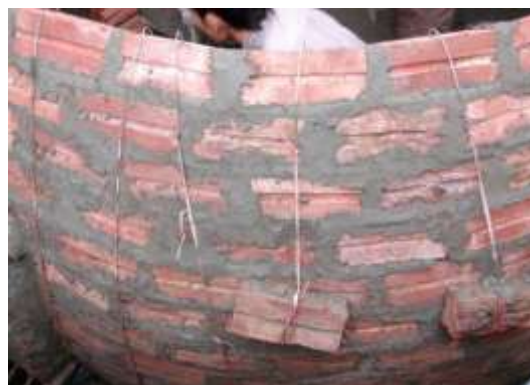
Figure 2.27. Keeping brick during vault construction
