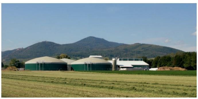
The Agrivalor waste-to-energy plant has its own hygienisation system with a capacity of 25,000 tonnes/year. More than 65 per cent of the thermal discharge is used to supply a nearby hotel with a casino.
