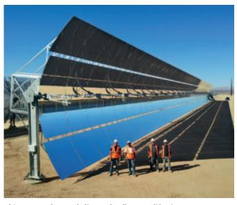
Ultimate Trough  $^{\scriptscriptstyle\mathsf{TM}}$  parabolic trough collector, California, USA.
