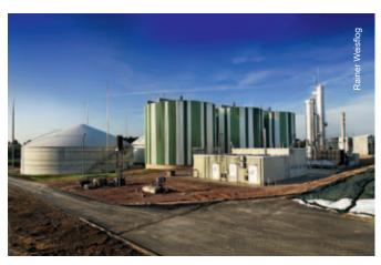
Naußlitz, Germany: This biogas plant, which started operation in 2011, can feed 700 Vn (standard cubic metres) of biogas per hour into the public gas grid.
