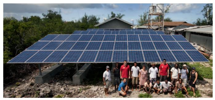
Aldabra, Seychelles: This hybrid PV plant with a peak capacity of 25.38 kilowatts (kWp) provides an autonomous energy supply for one of the research stations situated in the area.
