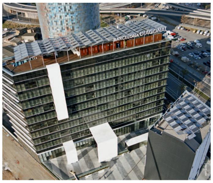
Barcelona, Spain: The ninety flat plate collectors installed on the roof of this hotel were made from environmentally friendly, single-variety materials which can easily be separated and recycled. The collectors used here have an expected life span of 20 years.
