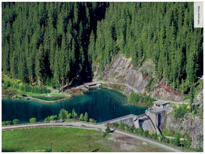
St. Anton, Austria: The Kartell storage power plant with a capacity of 4,239 kW makes use of water flowing from a drop height of 528 m at a rate of 0.90 m $^3/\text{sec}$ . The plant is run by two horizontal-axis, twin-nozzle Pelton turbines.
