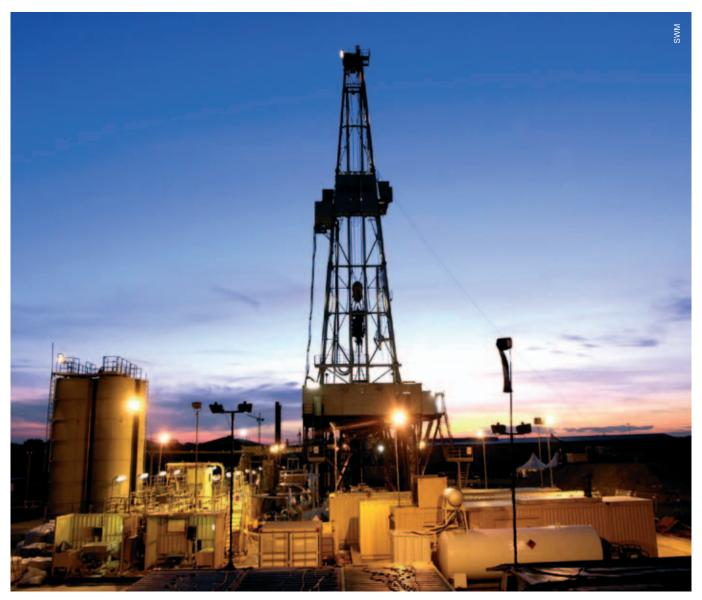
Sauerlach, Germany: The Sauerlach Geothermal CHP plant officially started operations in January 2014. The plant uses the roughly 140 °C thermal water both to provide heat for Sauerlach households as well as to generate electricity for around 16,000 households. This cuts annual emissions of  $CO_2$  by around 35,000 tonnes. The figure shows drilling work at the project site.
