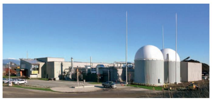
The illustration shows a biogas plant using two-stage dry-wet fermentation (GICON® Process) in Richmond, BC, Canada.
