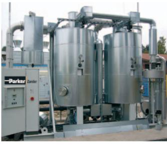
Regenerative, zero-loss adsorption system for drying Biomethane.
