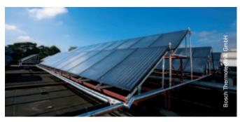
Hot water for the cafeteria of a Brazilian aircraft manufacturer is heated by the power from 180 flat plate collectors. The solar heat supports the washing and cleaning process in the commercial kitchen. The installation reduces the cafeteria's gas consumption by 69 per cent.
