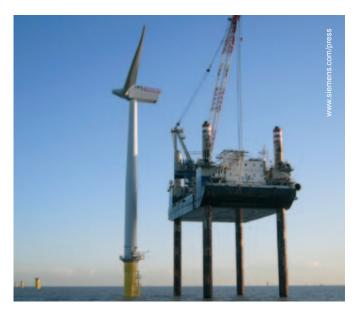
An installation vessel installing a wind turbine in the London Array wind energy plant.
