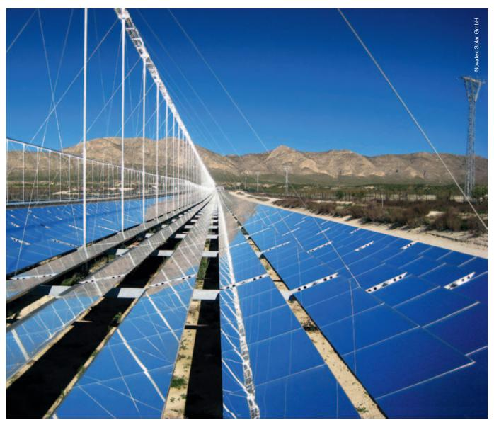
Murcia, Spain: The 30 MW Puerto Errado solar thermal power plant has been in commercial operation since August 2012. The power plant, with its 28 rows of linear Fresnel collectors, is the world's largest Fresnel solar power plant in operation. It produces 49 GWh of electricity per year, thereby saving 16,000 tonnes of  ${\rm CO_2}$  emissions. The energy generated here covers the needs of more than 12,000 households.
