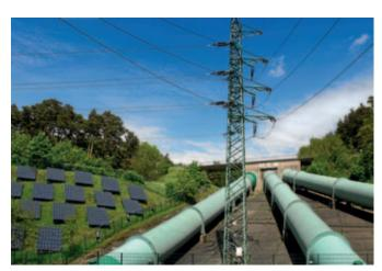
Geesthacht, Germany: The Geesthacht pump storage station on the Elbe River has been covering the electricity demand at times of peak load and as an emergency reserve in the event of blackouts since 1958. Renewable electric power from a 500 kW wind power plant and a 60 kW photovoltaic system pump the river water up a slope into an artificial reservoir.
