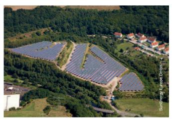
Unterbreizbach, Germany: Built on the ash heap of a coal-fired power plant, this solar park has a total capacity of 2.5 MWp and generates electric power for 750 households.
