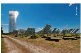
Jülich, Germany: From 2005 to 2010, the Jülich solar tower power plant was built as a solar-thermal operated water-to-steam power plant at a high temperature level. The plant has been used by the project partners for research purposes since 2011.
