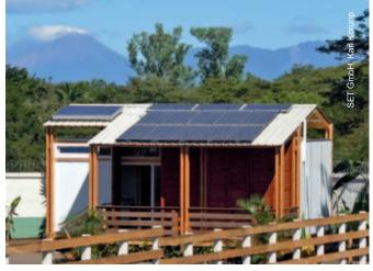
Léon, Nicaragua: The PV modules on the roof of this self-sufficient solar house provide electricity for a solar pump system, among other things. Solar-thermal collectors heat the process water.
