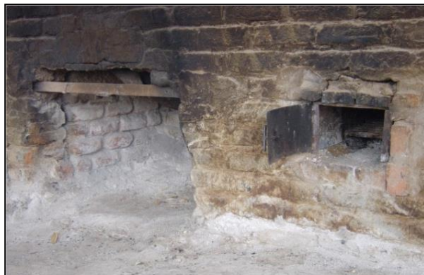
Figure 10: On right-hand side, an improved brick hearth system, Kaphuka Private Secondary School, Blantyre (note: improved hearth not used by cooks)
