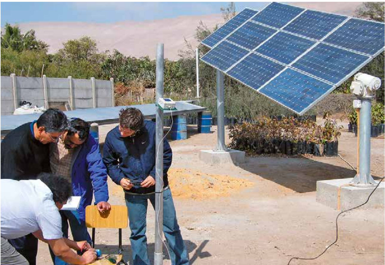
Figure 2.22: Performance test of solar generator
