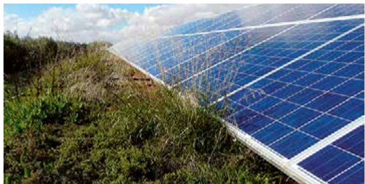
Figure 5.23: Example of shadowing by uncontrolled ground vegetation Source: GIZ / Andreas Hahn, 2015
