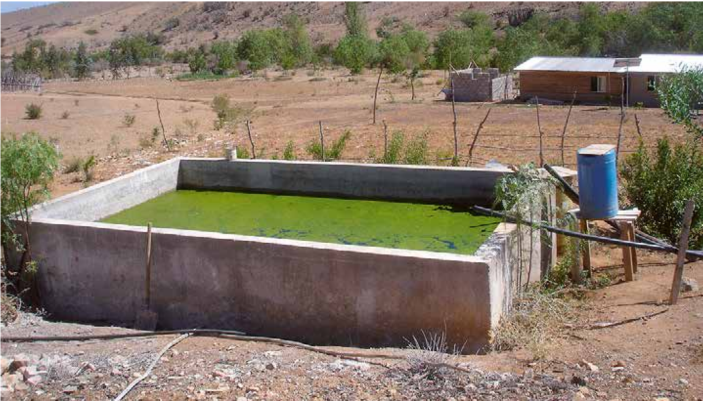
Figure 2.16: Example of an open water tank made of concrete in Chile
