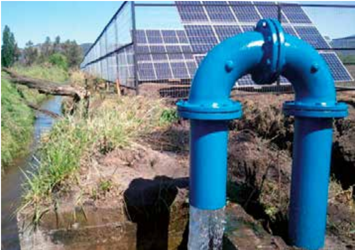
Figure 2.35: Lifting water to an upper reservoir in Chile Source: iEnergía Group, 2015
