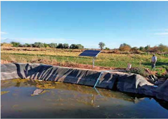
Figure 7.2: Reservoir filled by PV powered groundwater pump in La Tirana, Chile
