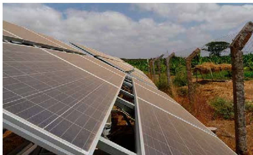
Figure 5.16: Shadowing of solar panels by fence in Kenya
