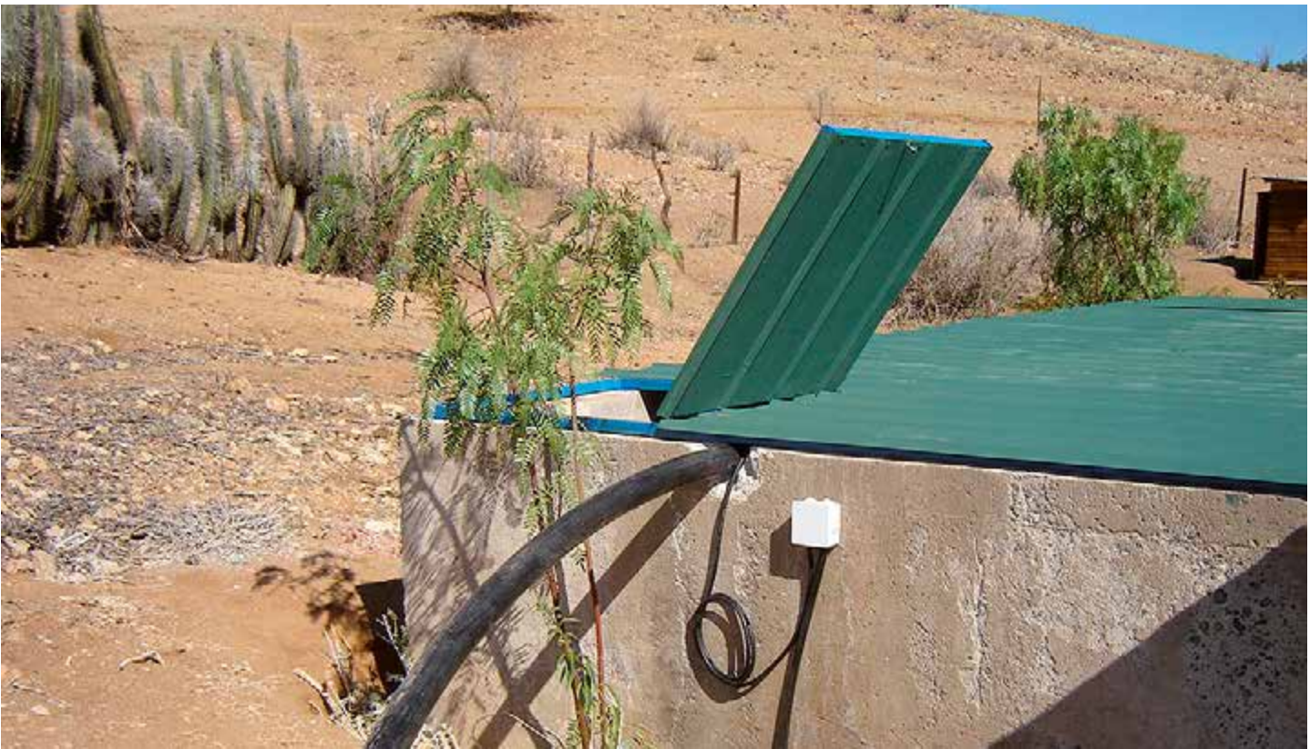
Figure 2.17: Concrete tank covered with a metal lid
