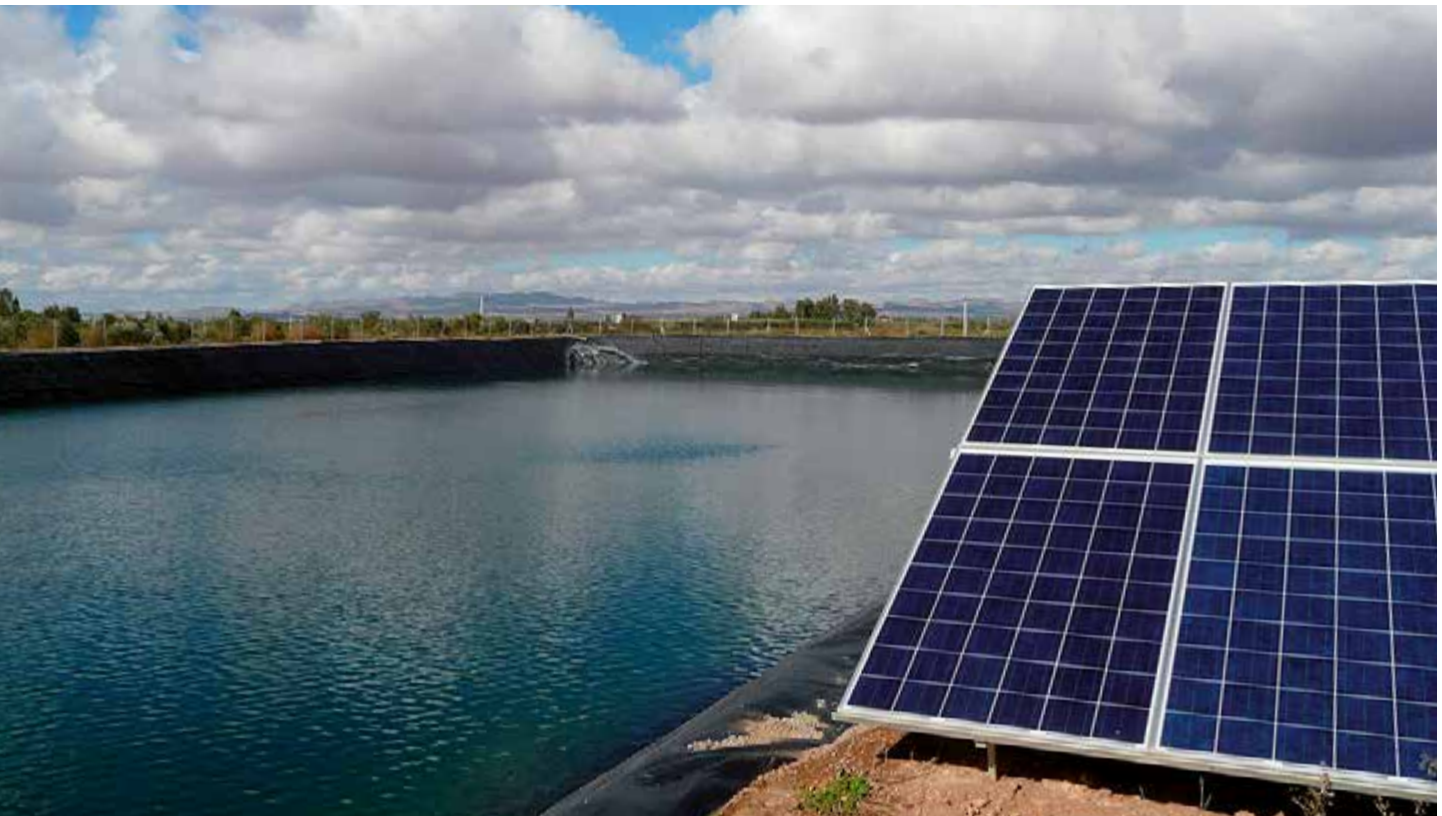
Figure 2.15: Example of an open plastic foil-lined reservoir often used in Morocco
