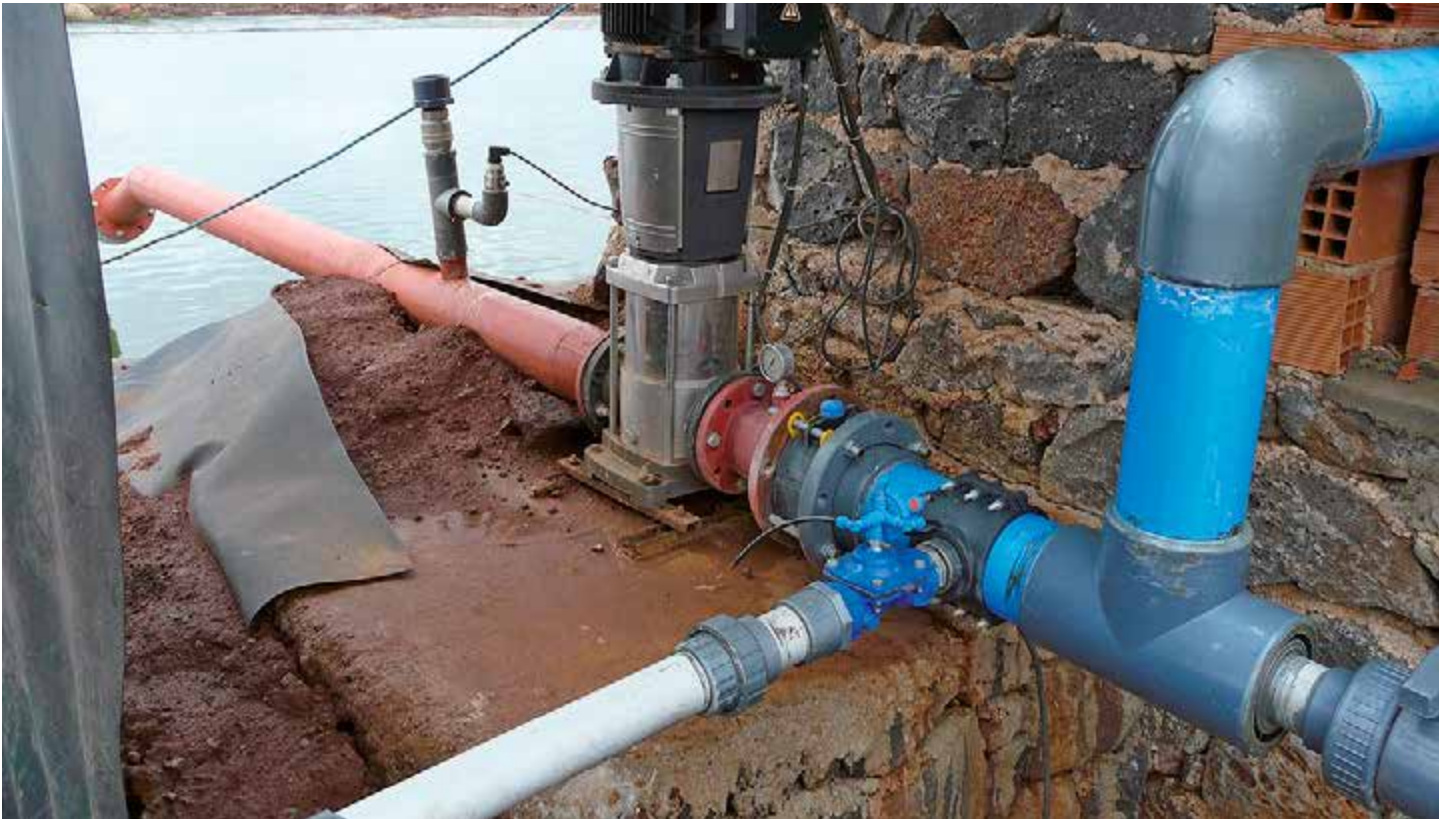
Figure 2.13: Surface-mounted single-stage centrifugal pump with AC motor
