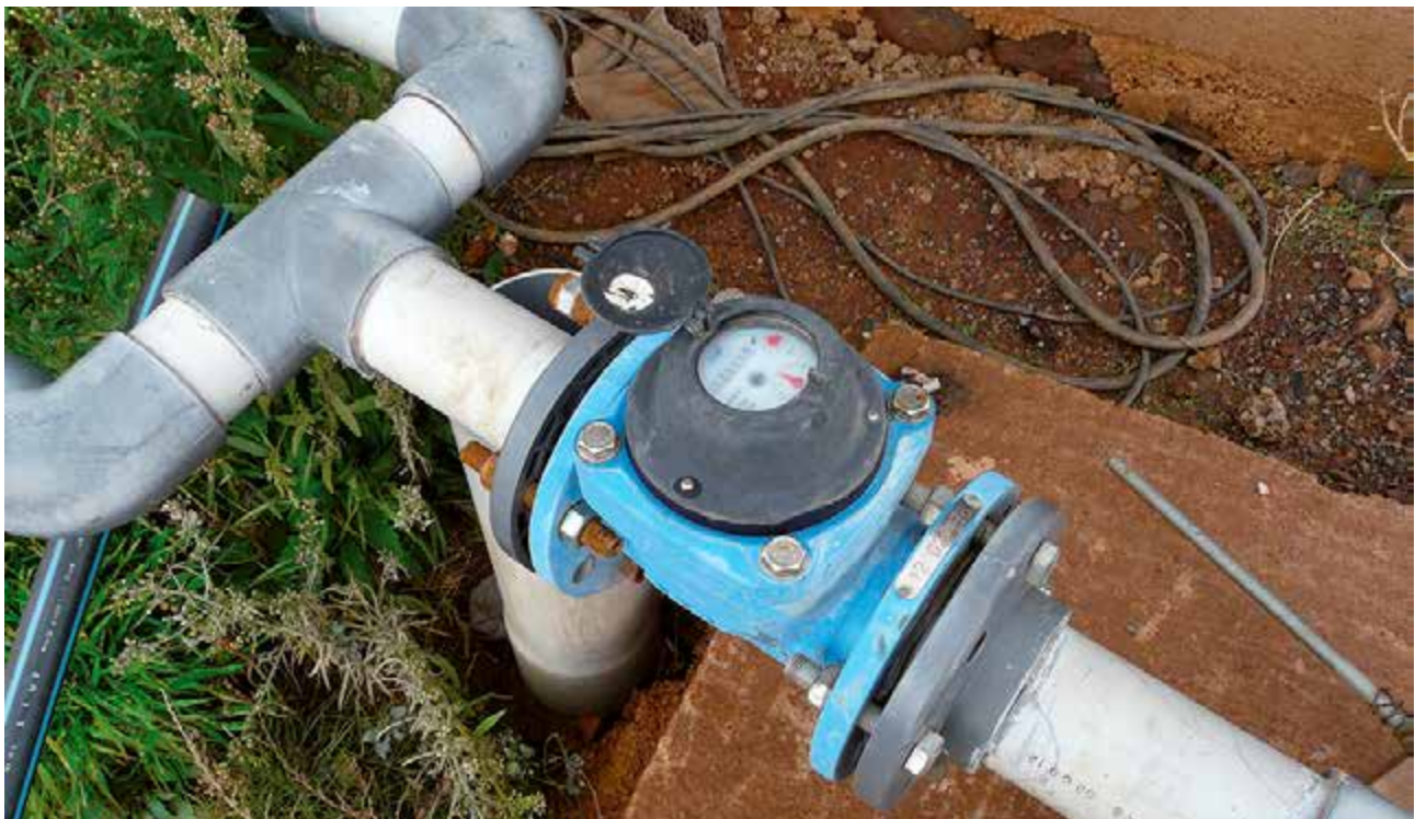
Figure 8.11: Water metering device – an essential but rare component of SPIS
