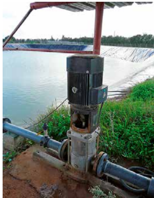
Figure 2.34: High performance AC surface pump with fertiliser injection valve
