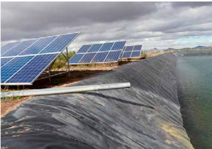
Figure 2.36: Combination of submersible and surface pump in Morocco Source: GIZ / Andreas Hahn, 2015
