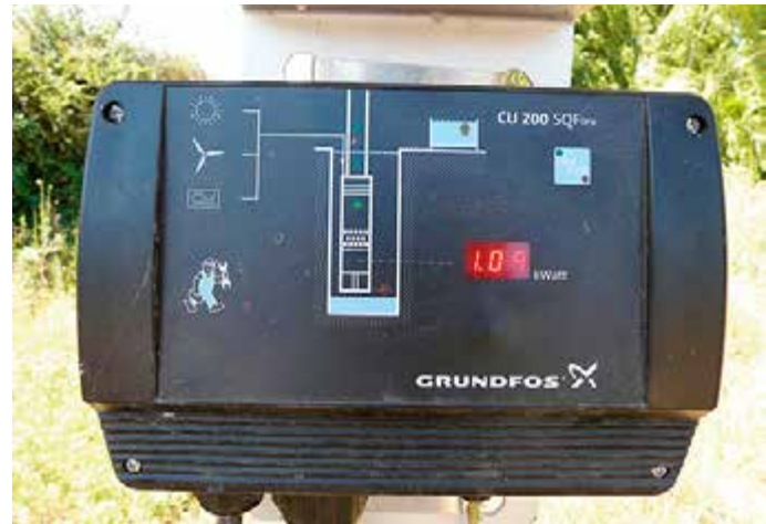
Figure 2.8: Pump controller with display and LED fault indicators
