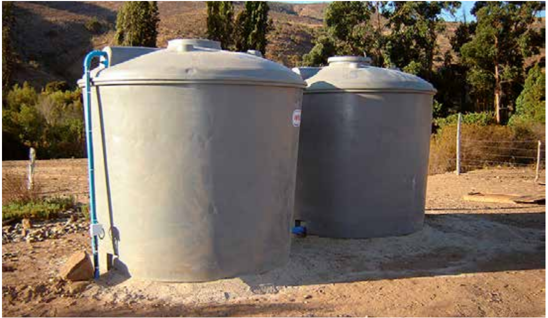
Figure 2.18: Example of relatively inexpensive plastic tanks
