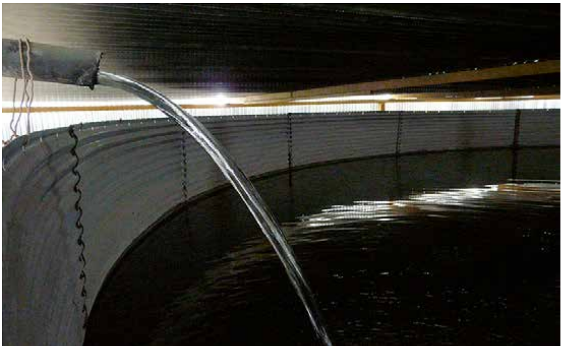
Figure 2.19: Example of a large water storage tank made of corrugated iron sheet in Chile
