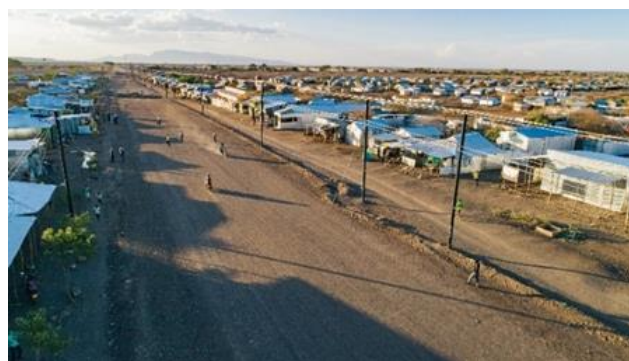
Households, businesses and institutions connected to electricity supply from Kalobeyei settlement mini grid. © GIZ Kenya, 2022
