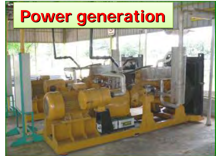
Modified gas engine
