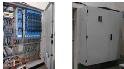
Figure 188: AC connection unit for a large-scale solar power system
