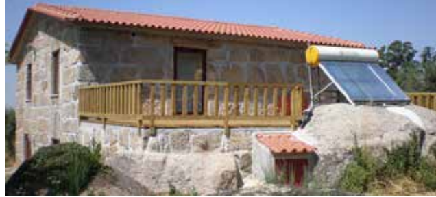
Figure 44: SWH – open system
