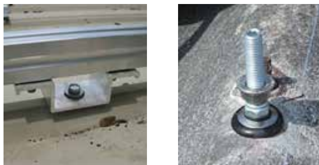
Figure 169: Support solutions for roof parallel installation
