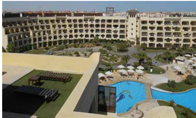
Figure 57: Large hotel unit in Hurghada, Egypt
