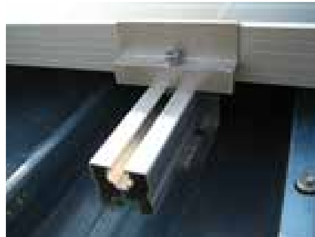
Figure 170: Standard module fasteners
