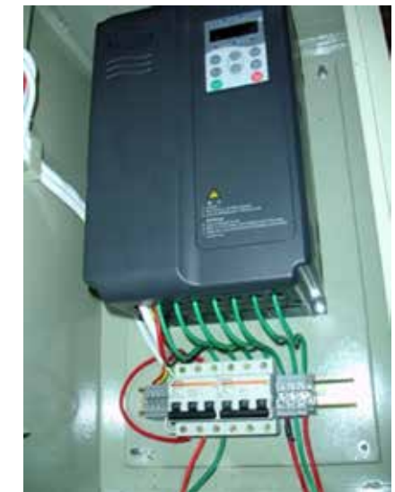
Figure 27: Solar Pump Inverter for direct connection to a motor
