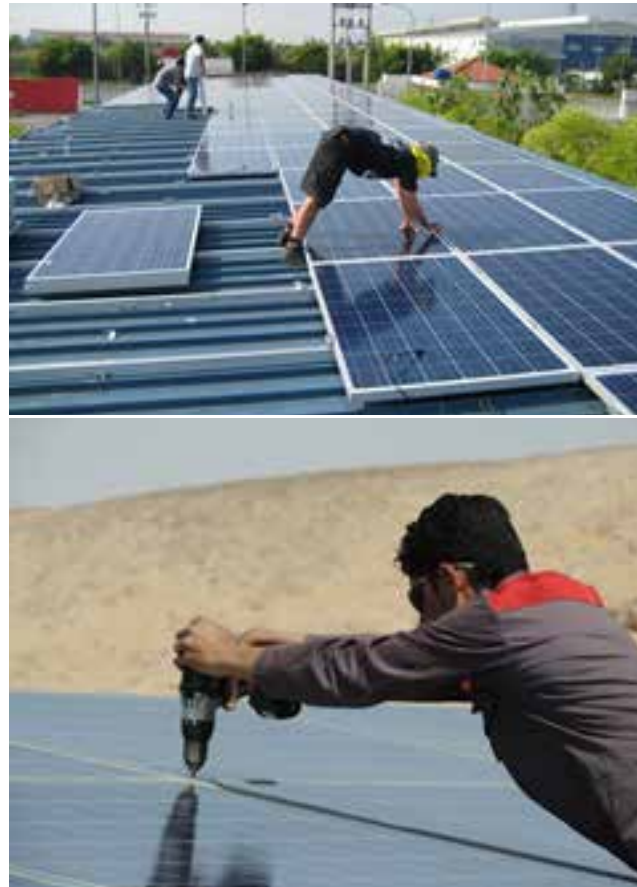
Figure 214: Assembly of PV panels
