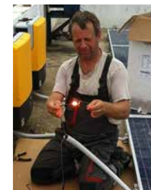
Figure 210: High DC voltage in the string wiring, if wire endings are free and strings are connected.
