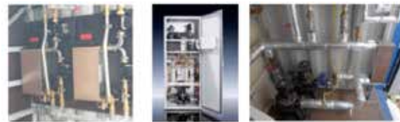
Figure 249: Pre-assembled module to transfer the heat to the storage
