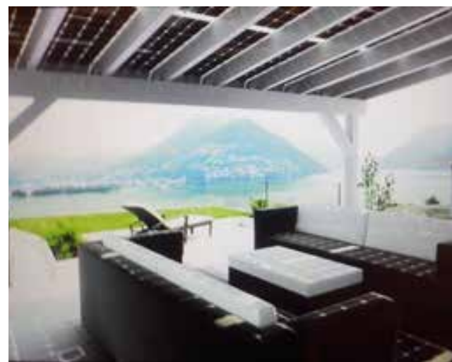
Figure 176: Sun terrace covered with semi-transparent glass-glass modules for shading and power generation
