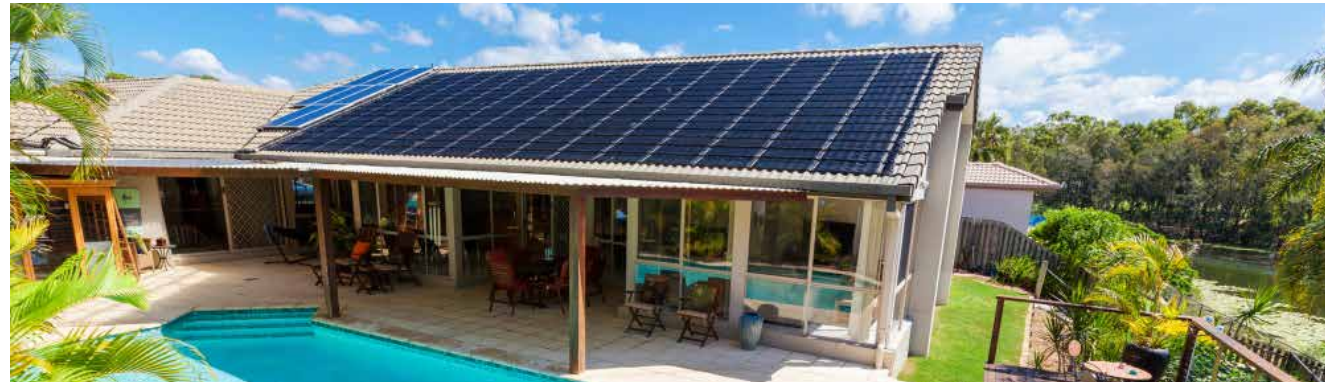
Figure 63: Solar thermal system as a highlight in front of the hotel
