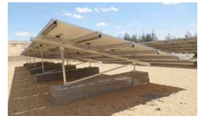
Figure 173: Solar on-ground installation with concrete foundations in Bahariya, Egypt
