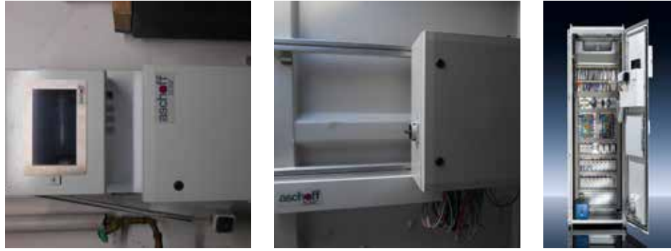
Figure 247: Control unit of a solar thermal system – pre-assembled in a control box
