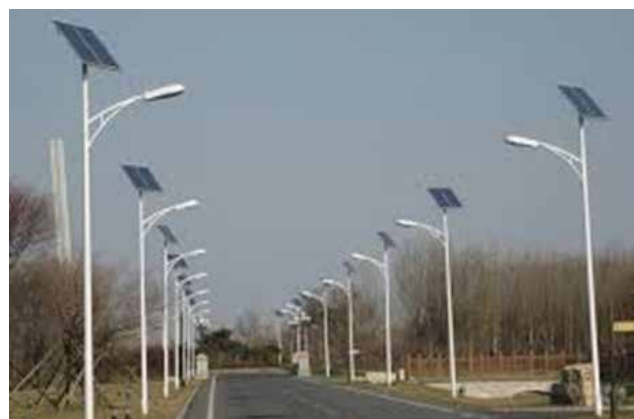
Figure 81: solar streetlight and fountain pump
