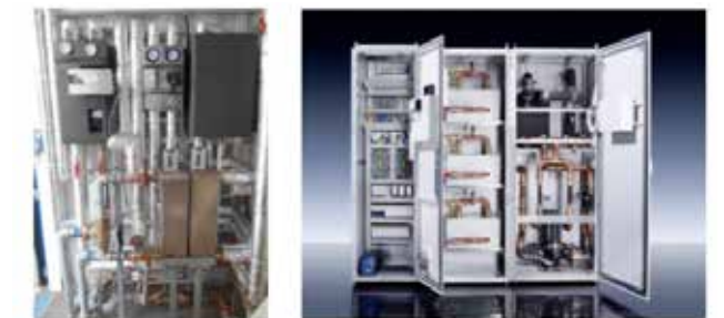
Figure 246: Pre-assembled complete solar thermal system with solar command (e.g. controlling module), drive module (e.g. pump module) and interface module (e.g. transfer unit)
