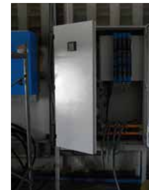
Figure 209: Installation of an AC connection unit
