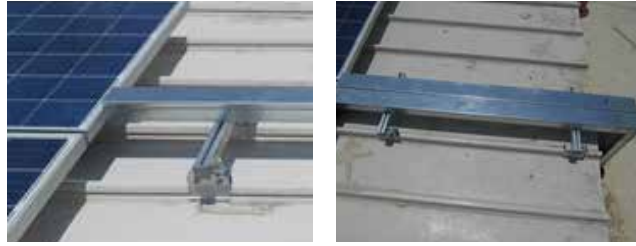
Figure 179: Wire protection via cable ducts
