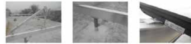
Figure 250: Support structure for a flat roof
