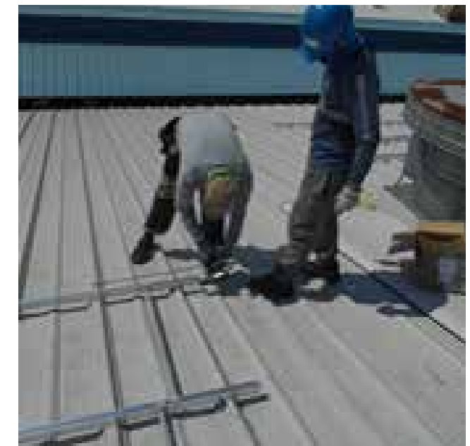
Figure 203: Baseline for the support structure
