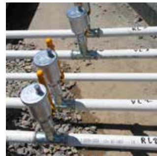
Figure 257: Air bleeder
