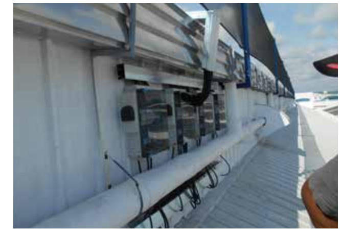
Figure 211: Installation of DC string combiner boxes
