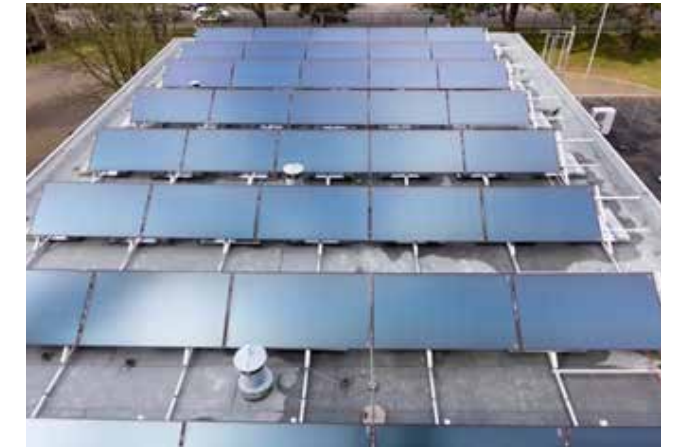
Figure 61: flat roof installation of a solar thermal system
