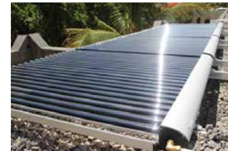
Figure 278: Evacuated tube collectors or hermetic sealed flat plate collectors to prevent from
