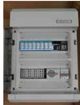
Figure 187: AC connection unit for a small size solar power system
