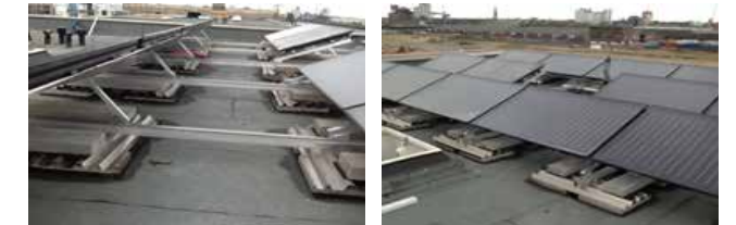
Figure 223: Roof top support structures
