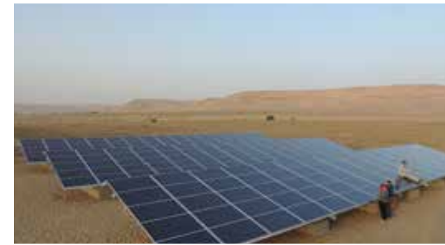
Figure 215: Installation of solar panels
