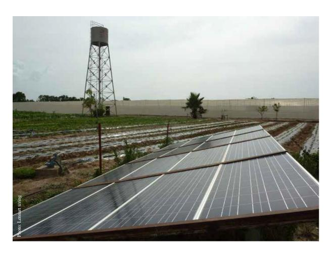
SPIS with an elevated reservoir used for irrigation in- and outside of the greenhouse (Source: Lennart Woltering)
