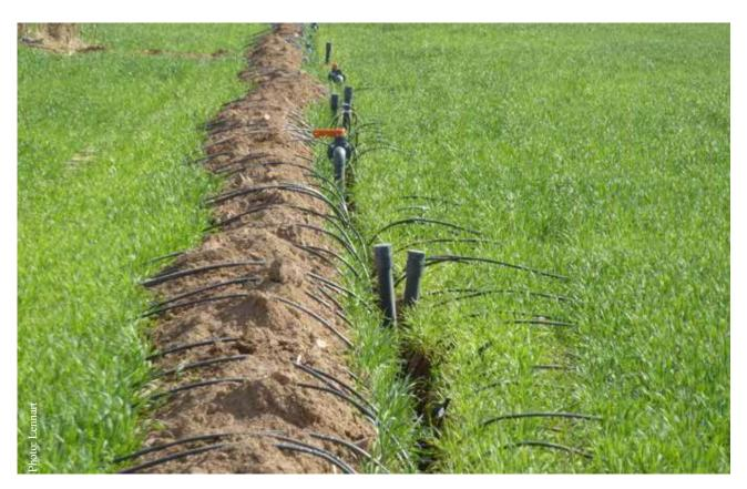
Installation of a drip irrigation system (Source: Lennart Woltering)
