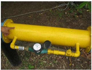
Water metering of source water with a low-cost proportional water meter
