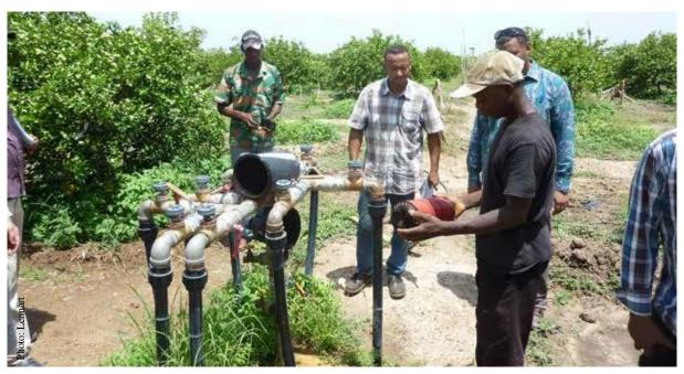
Irrigation head with a disc filter and multiple valves that guide the water to different sections of the irrigation system (Source: Lennart Woltering).
