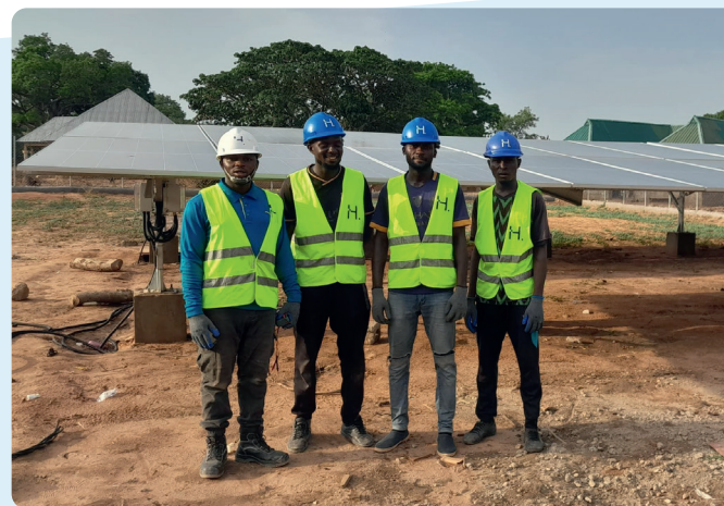
Figure 3. Installation of one of the mini grids (Source: Husk Power Systems)
