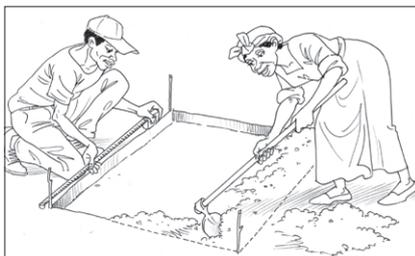
**1.2** Pour mixture of clay( with chopped grass or sawdust) into the dug-out foundation area and compact it firmly.
