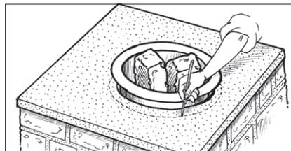
**7.3** Scoop out the excess clay mixture inside the line, going down to the level of the pot rests.
