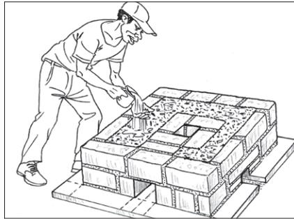
**4.4** Ensure the surface is even and horizontal by using a spirit level and tape measure.
