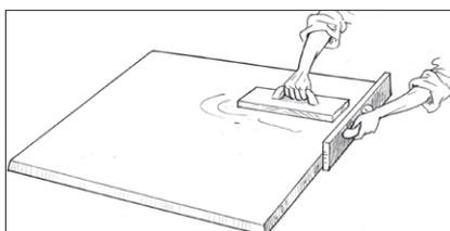
**1.5** Mark the midpoint of each side of the slab and draw lines to join opposite sides. Where the lines cross is the centre of the combustion chamber — mark it with a stick. From the centre, work outwards to make your other measurements. Refer to the stove plan on page 5.
