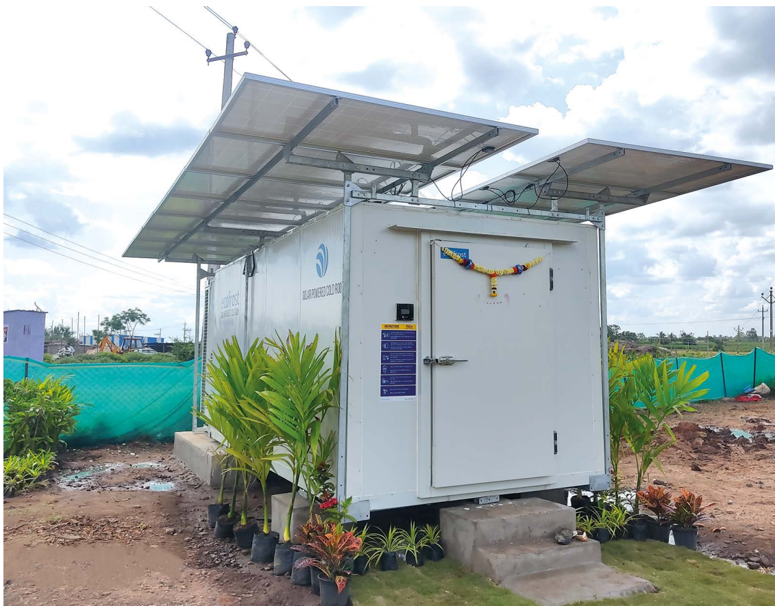
Figure 5.14 Attached solar array ( Ecofrost ).
