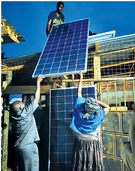
Figure 6.8 PV modules installation ( Solar Cooling Engineering ).
