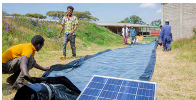
Picture 1: Installation of a solar dryer at one of the beneficiary cooperative premises
