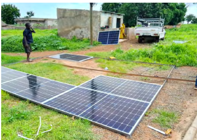
Figure 2: Solar panel installation
