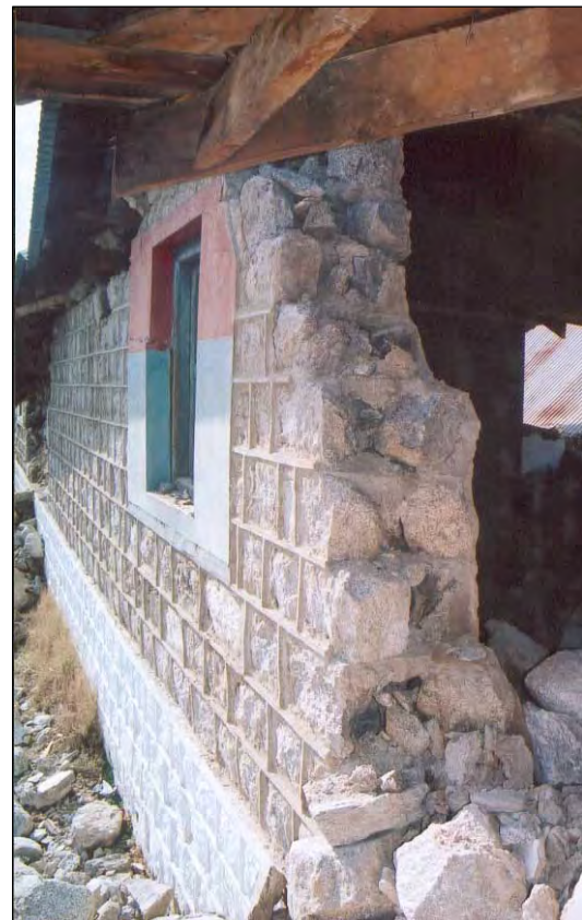
EXAMPLE OF POLICE POST WITH CUT-FACE STONE WALLS AFTER AN EARTHQUAKE
