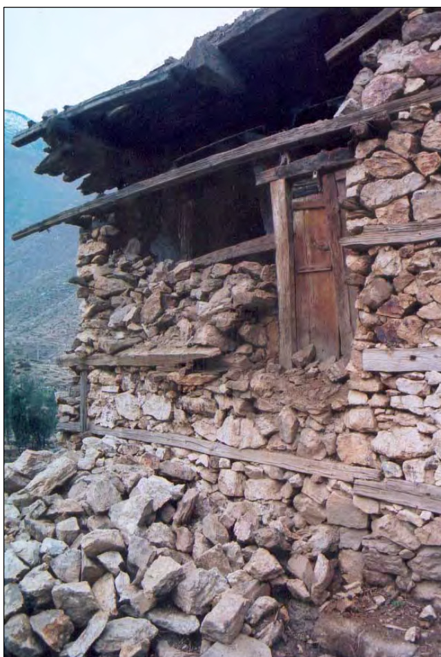
OLD BUILDING WITH TRADITIONAL WOODEN TIE BEAMS
