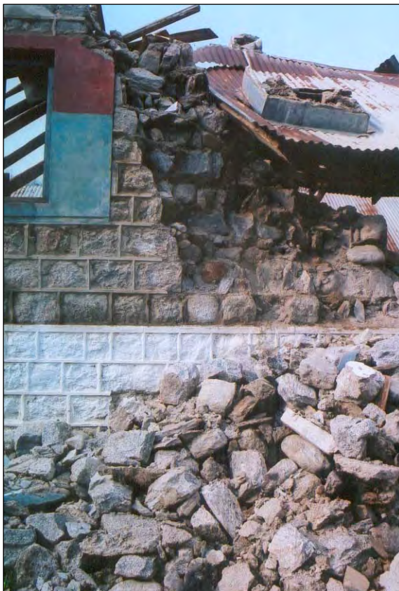
EXAMPLE OF POLICE POST WITH CUT-FACE STONE WALLS AFTER AN EARTHQUAKE
