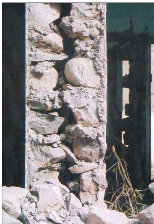
PHOTO LEFT: CROSS-SECTION OF TRADITIONAL WALL SHOWING LACK OF BONDING BETWEEN FACES, BUT WITH THE USE OF A LARGE AMOUNT OF CEMENT MORTAR AND PLASTER. PHOTO RIGHT: TRADITIONAL WALL, THE TOP IS HELD IN PLACE BY THE ROOF.
