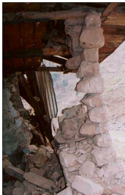
PHOTO LEFT: CROSS-SECTION OF TRADITIONAL WALL SHOWING LACK OF BONDING BETWEEN FACES, BUT WITH THE USE OF A LARGE AMOUNT OF CEMENT MORTAR AND PLASTER. PHOTO RIGHT: TRADITIONAL WALL, THE TOP IS HELD IN PLACE BY THE ROOF.
