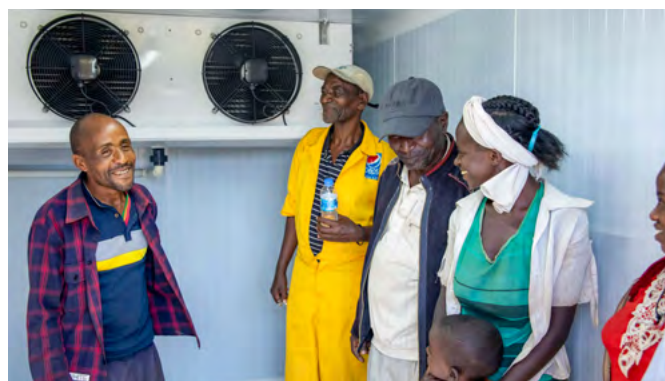
Picture 3: Inside the Cooling Container
