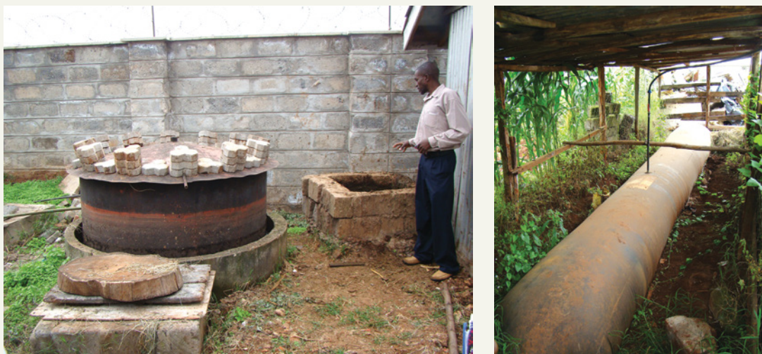
FIGURE 2.19. Small on-farm anaerobic digester in Kenya using manure from a 4 cow dairy herd with butanol gas storage bag.
