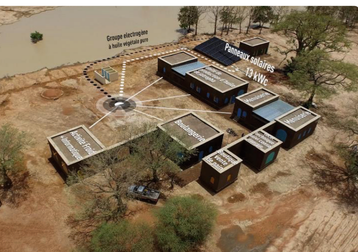
Figure 2. Air view of GBA electricity supply system and premises (Source: GERES)
