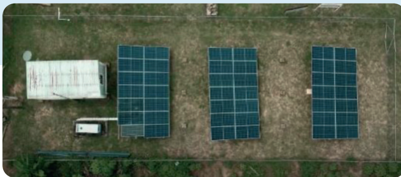
Figure 1. Generation system of Prado Power’s 20 kW mini grid in the Mbiabet Ikot Esieyere community. Source: RMI, 2024a.
