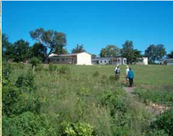
Some of the buildings of the EPF school at Bilibiza
