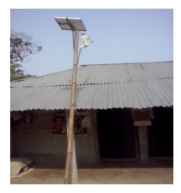
➤Two LEDs of 2.4 W (~200 lumens and 7-8 lux from a height of 2.5 metre) and a mobile charging point
