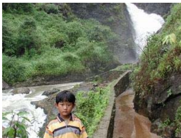
Power for the future: Young inhabitant stands at the head race channel of an 80 kW MHP
