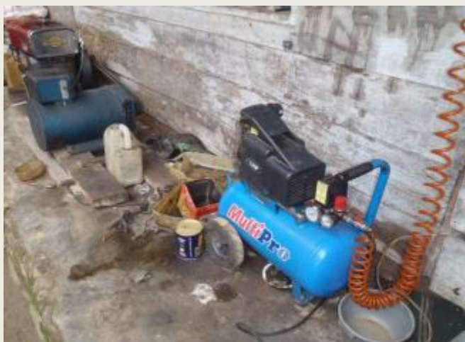
Figure 28 Diesel genset for PUE
