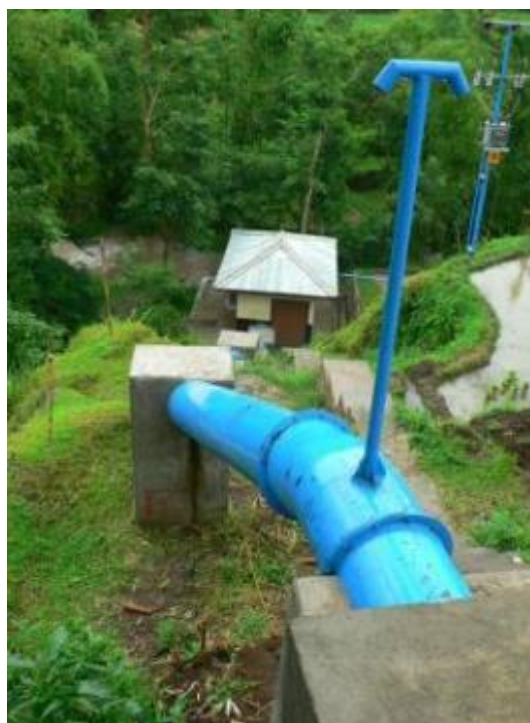
Figure 10 From head to the powerhouse
