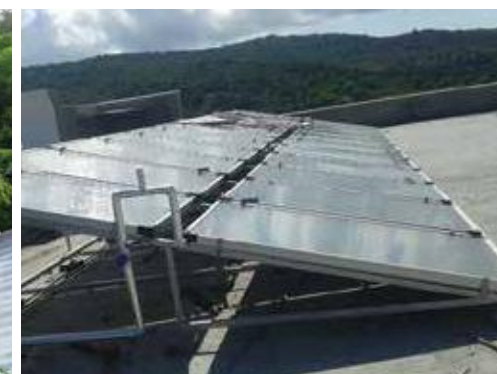
SOLAR WATER HEATING SYSTEMS – THIEN THANH HOTEL, PHU QUOC ISLAND Capacity: 13.000 L
