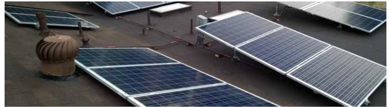
Capacity: 5.5 kWp Estimated lifetime production: 15.7 MWh
