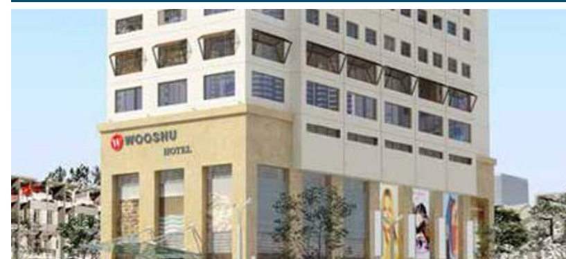
WOOSHU COMPLEX PROJECT – BIEN HOA CITY, DONG NAI PROVINCE
