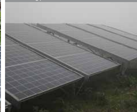
Eden resort project – Phu Quoc island, Kien Giang province
