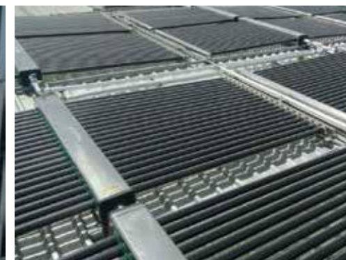
SOLAR WATER HEATING SYSTEMS – SOUTH VINA CO. LTD Capacity: 20.000 L
