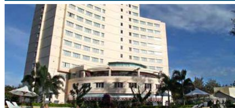
PARK DIAMOND HOTEL PROJECT – PHAN THIET CITY, BINH THUAN PROVINCE
