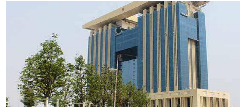
BINH DUONG ADMINISTRATIVE BUILDING PROJECT – BINH DUONG CITY
