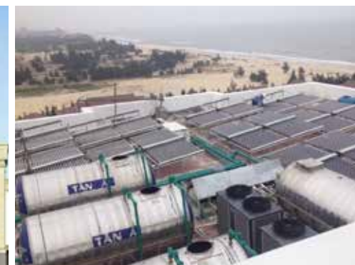
SOLAR WATER HEATING SYSTEMS – GOLD COAST HOTEL RESORT & SPA, QUANG BINH PROVINCE Capacity: 12.000 L
