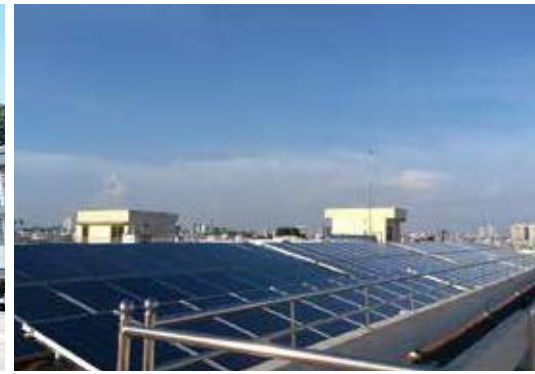
Grid-tie power system of 160kWp (Phase 1)
