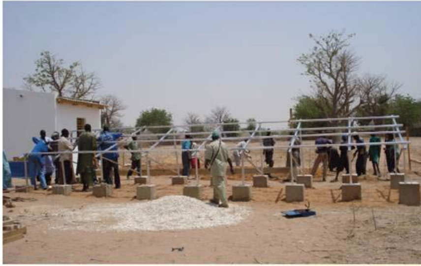
Construction of support structures
