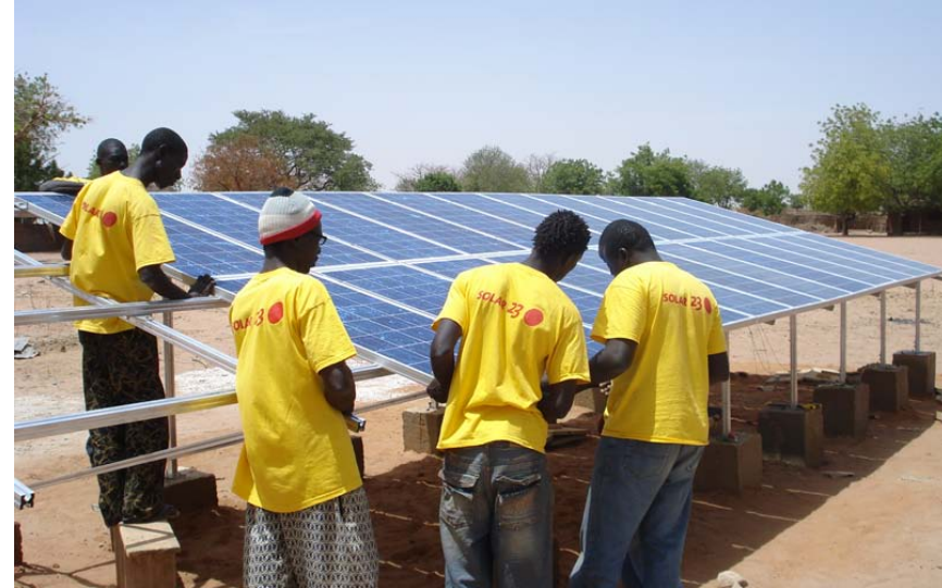
Positioning and assembling of modules
