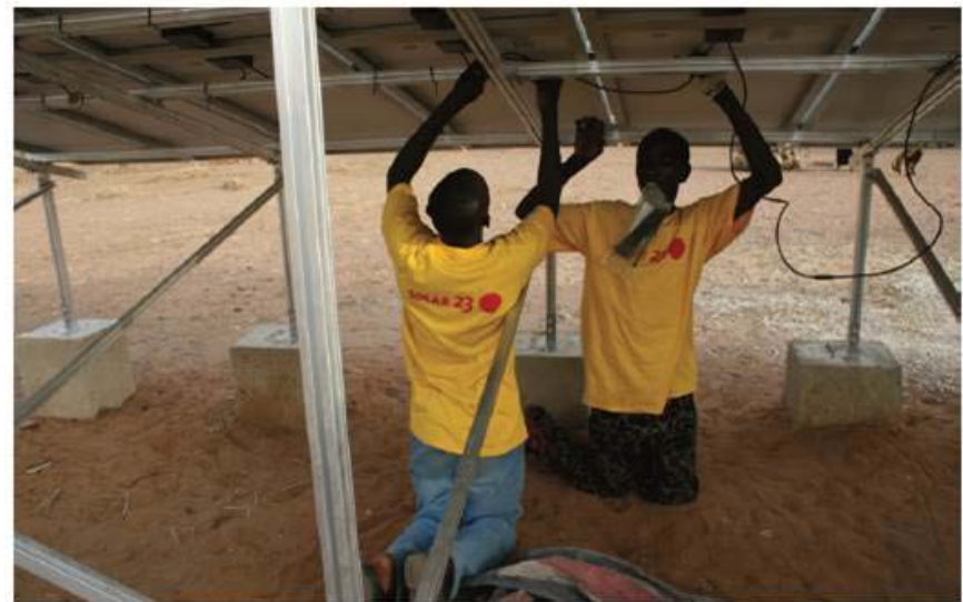
Cabling of modules
