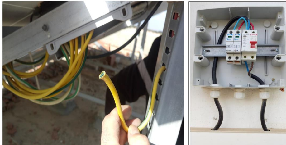
Figure 52: inexistence de la MALT
