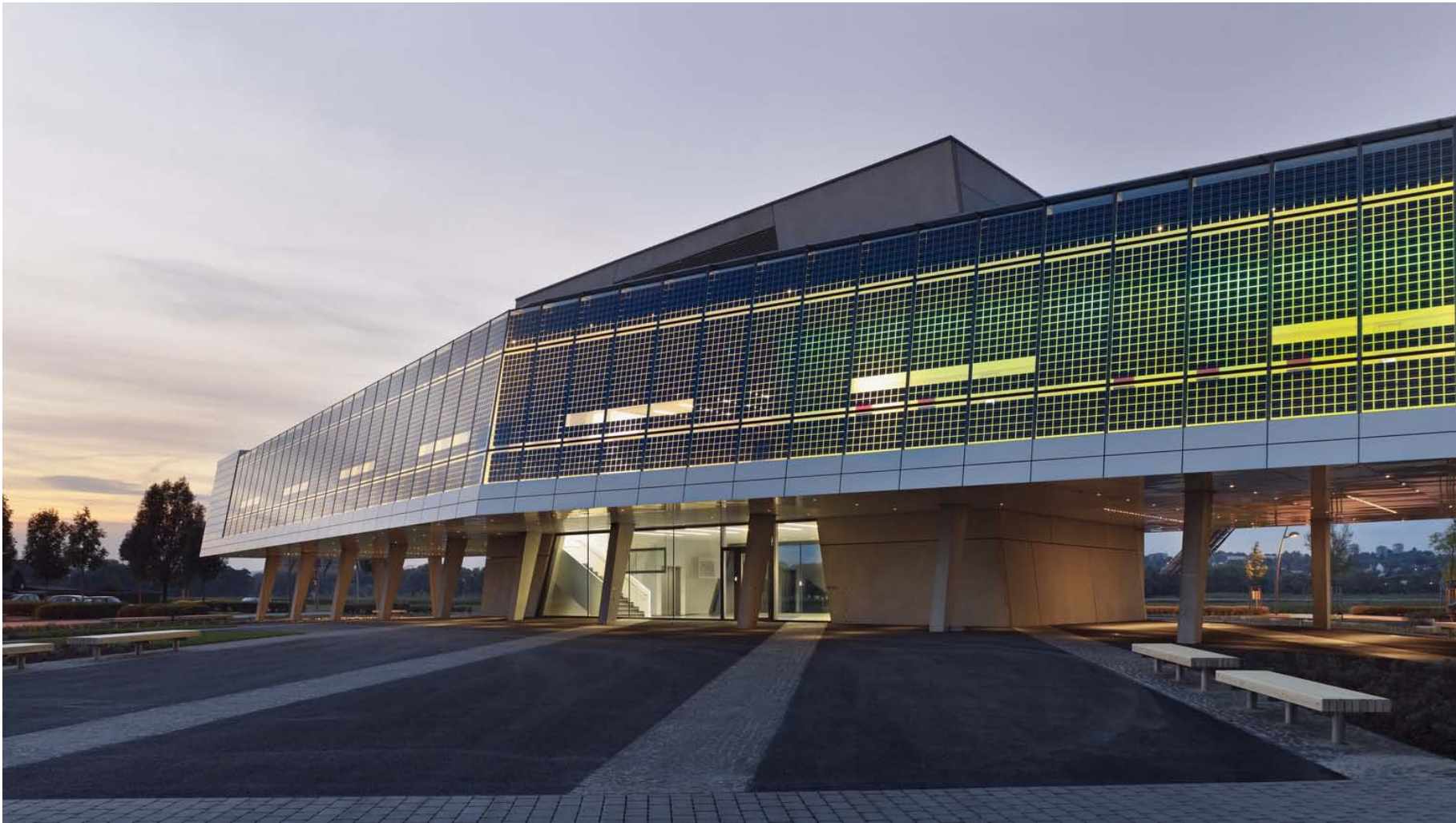
Picture: Off-Grid Building in Niestetal/Germany „SMA Solar Academy“
