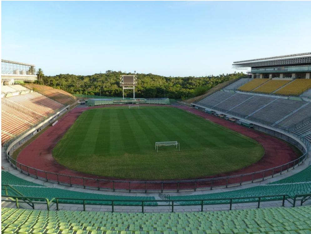
Figure 27: View of the entire stadium from the north.
