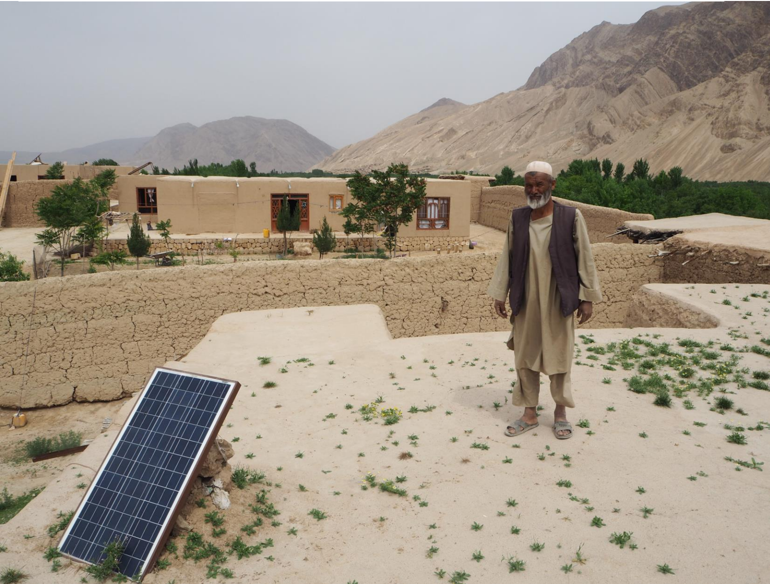
Figure 1 Talkhaki, Samangan: A research participant stands with his solitary solar panel. It charges a battery which powers light bulbs and mobile phone charging.
