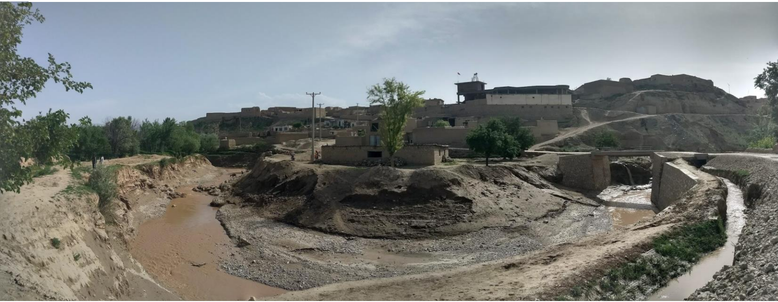
Figure 15 Dalkhaki village, Samangen: electricity poles without transmission lines stretch along the road
